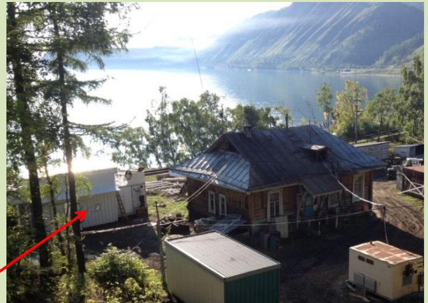
Operating Shore Station
