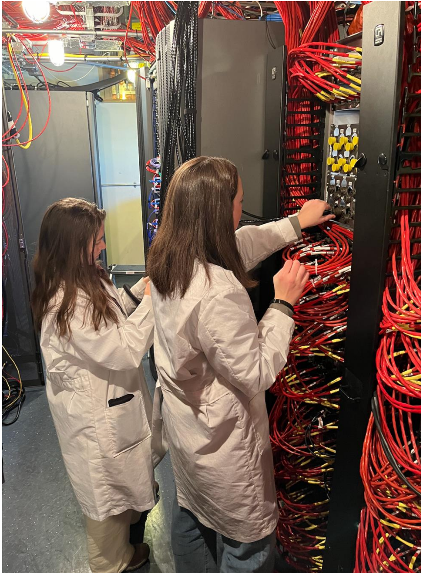
A. Bishop and K. DeHolton installing patch cables from the Upgrade surface cables to the FieldHubs (24–25)
