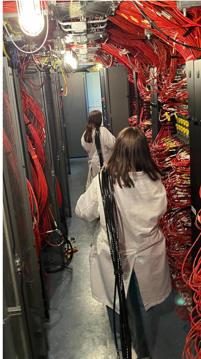
A. Bishop and K. DeHolton installing patch cables from the Upgrade surface cables to the FieldHubs (24–25)
