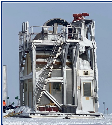
Installation of 6 strings at South Pole in 2026
