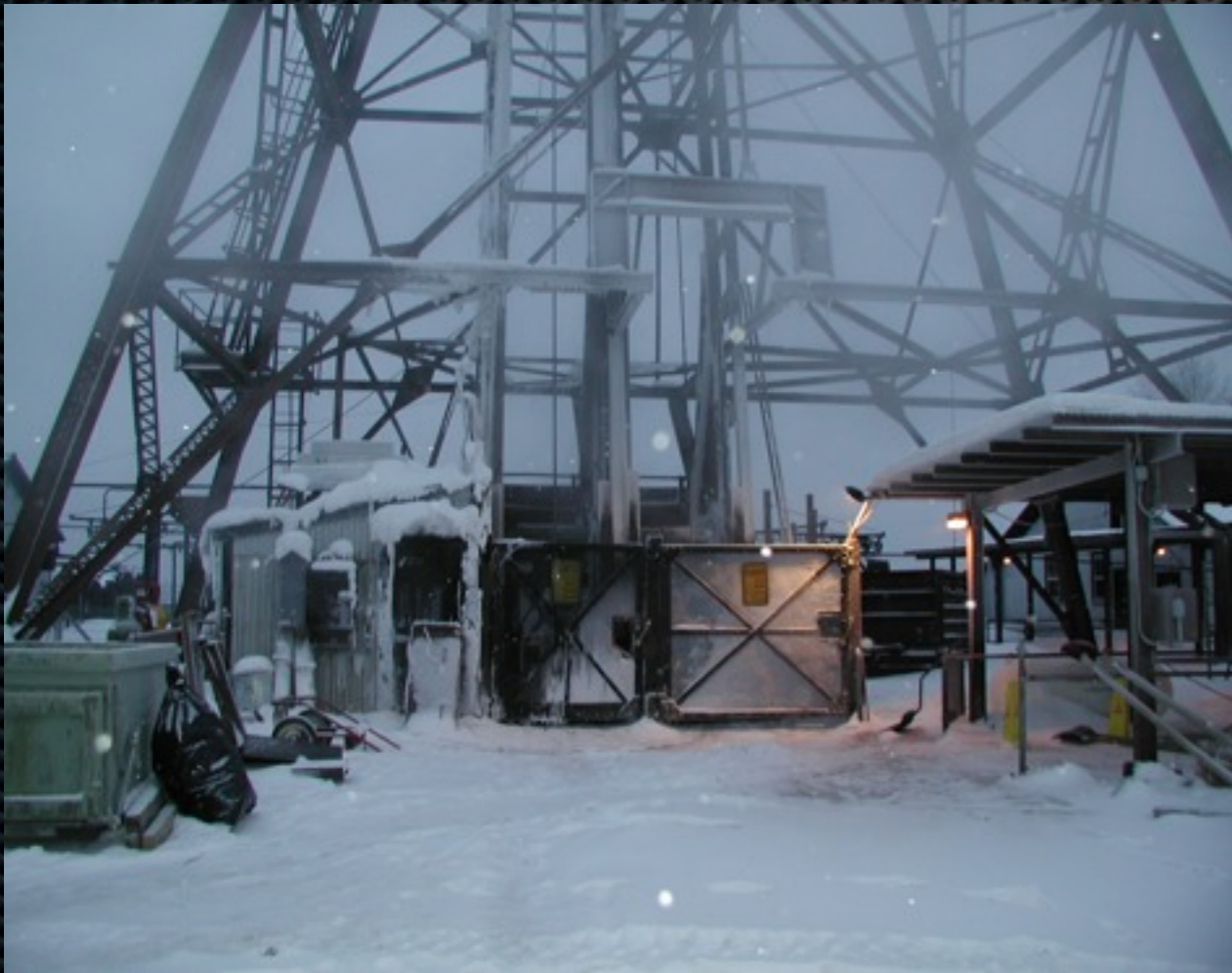
Entrance to the mine
