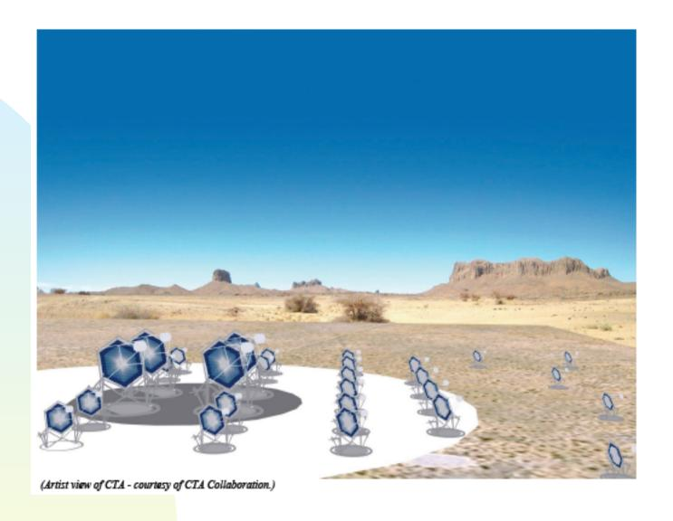
A TYPICAL ARRAY FOR THE SOUTHERN SITE: 4 large telescopes of 23mØ each, 35 telescopes Of 12 mØ, 60 telescopes of 6 mØ each, distributed over 1–2(5) km\*\*2. Likely site: Namibia or Argentina or Chile
