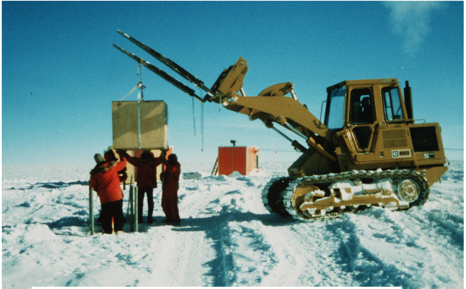
Lifting a SPASE scintillator box into position: November 1987
