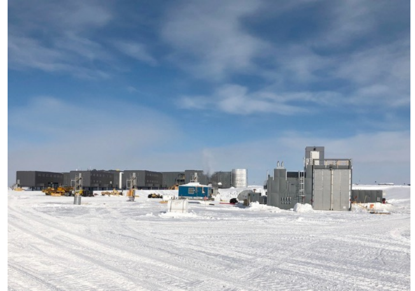
Gen2 Phase 1 (Upgrade) drill camp; January 29, 2020
