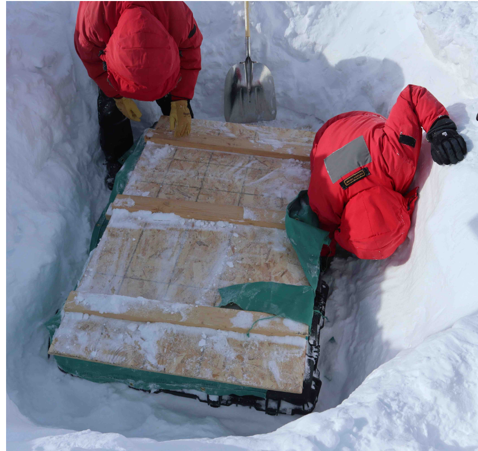
excavation in 2019 for radio upgrade
